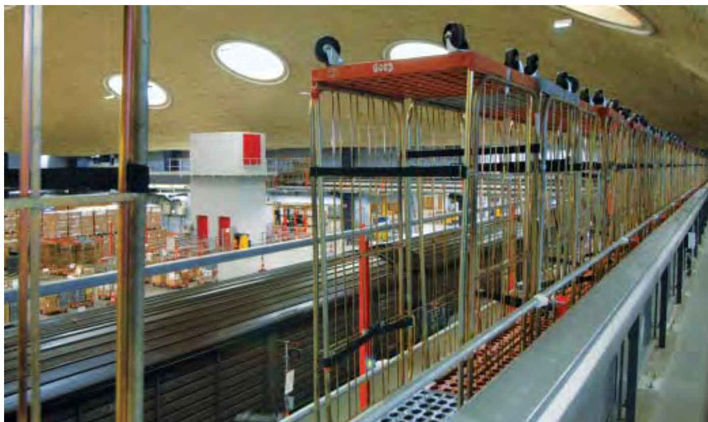
The buffered wheelcontainers wait on the upper level for their distribution to the individual conveyor routes.
