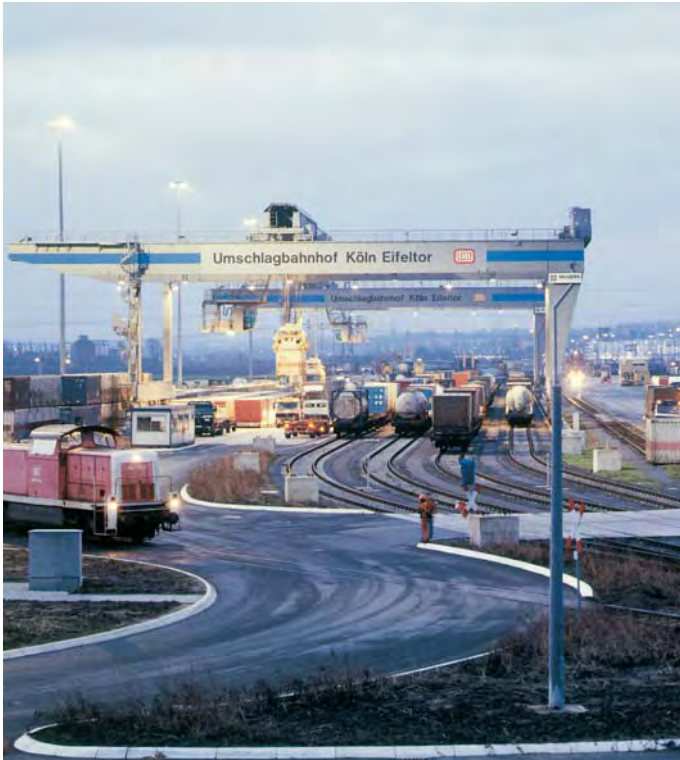
The problem of cable capacitance with long control cables also often occurs in large-scale installations such as with crane systems in container terminals.
